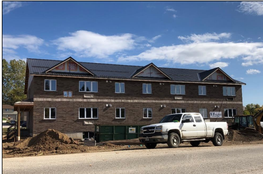
Figure 2: Durham Housing Build under Construction
