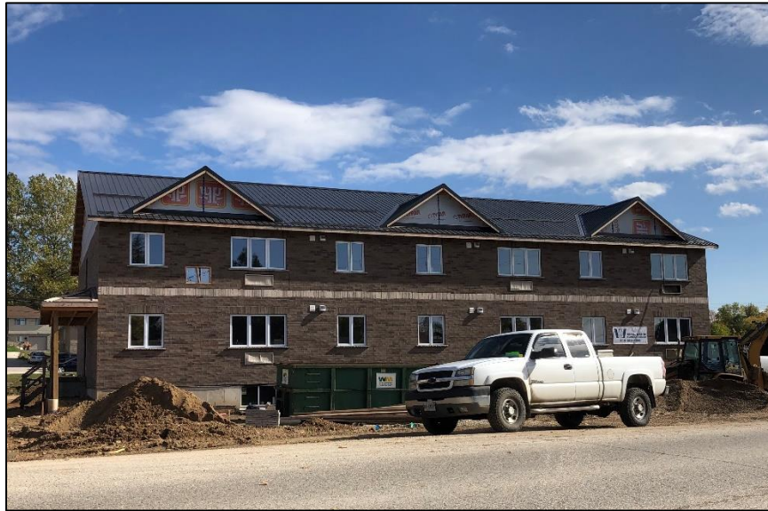
Figure 2: Durham Housing Build under Construction
