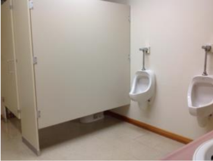
Inside Accessible Washroom:
